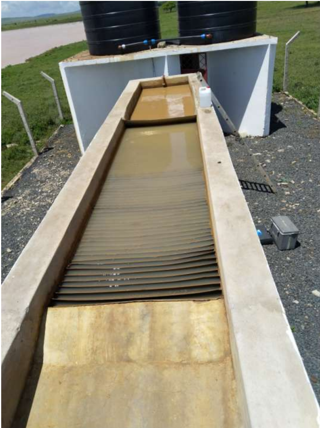
Figure 7.22: Pilot Lamella Settler installed at Nadosoito, in Monduli district, Tanzania for Dam water treatment (Courtesy, K. Njau, 2020).
