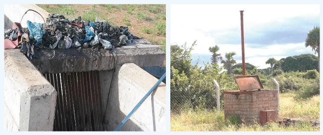
Figure 4-8: Solid waste collected at bar screen (left) and a typical incinerator (burning chamber) (right)-Kahama
