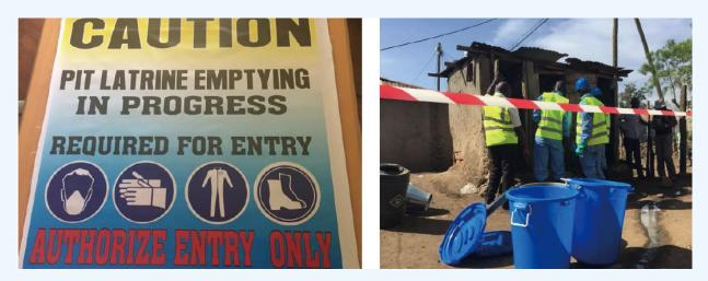
Figure 4- 6: Sample hazardous workspace signage (Left), Barrier tape erected around workspace (right).
