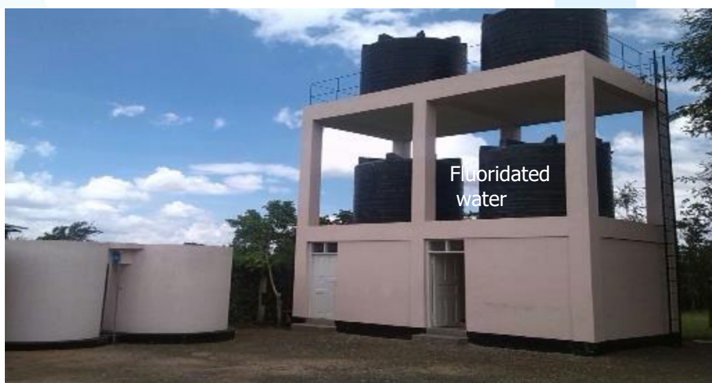
Figure 3-20: Mwendo Community Defluoridation Plant
