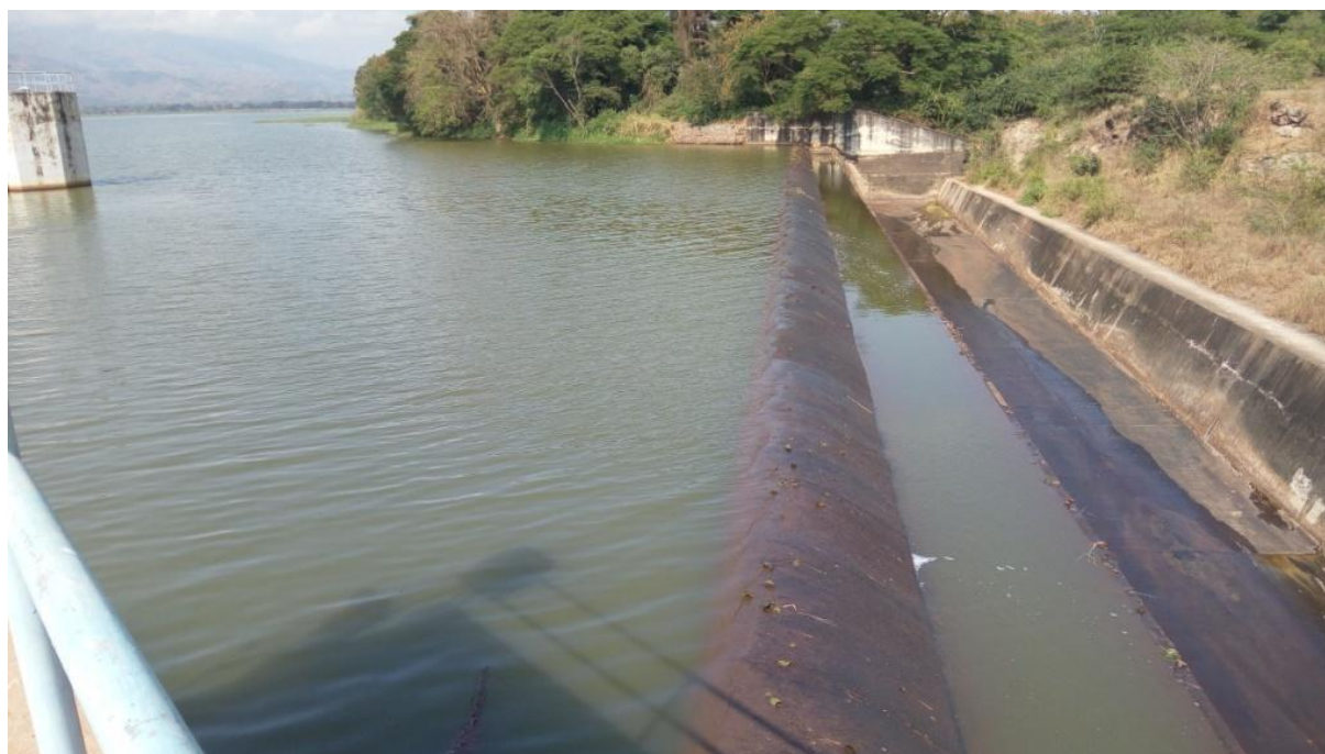
Photo No. 1: Mindu Dam
