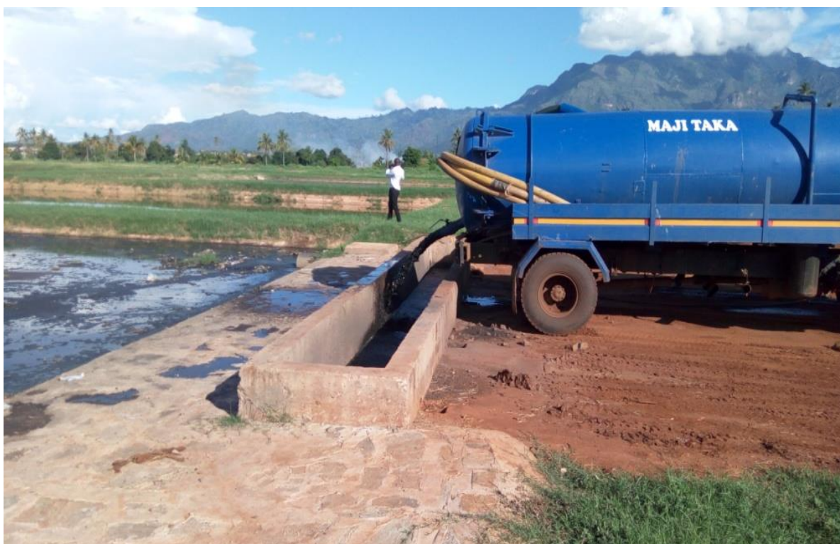
Photo No. 4: Wastewater disposal at Mafisa Waste Stabilization Ponds from unconnected individuals
