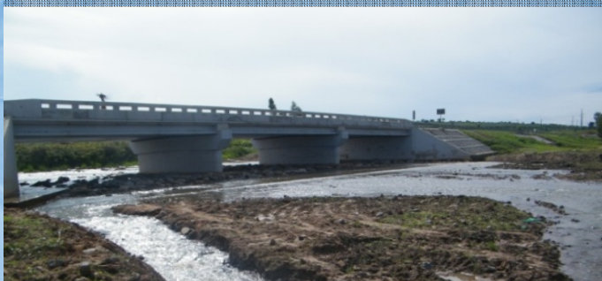
Lwiche River Mpanda Road Bridge
