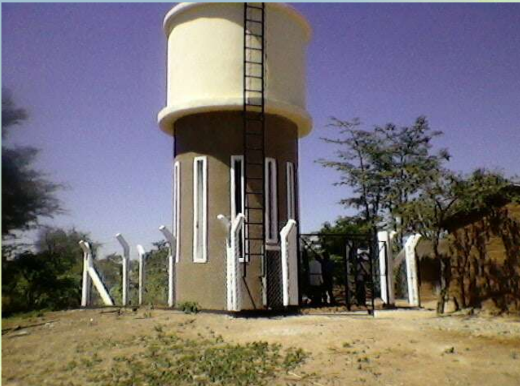
The completed raiser tank constructed under WSDP financing at Chela Village in Kahama District, Shinyanga Region
